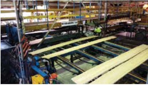
• Edger Operation with new operator console and added panel view HMI
