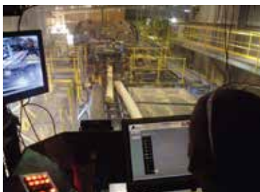
• SA Pine Kuitpo Operator Booth (where scanner is installed)
