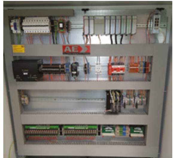
• PICTURED: Updated Networks using an Allen Bradley CompactLogix PLC with Delta Motion control
